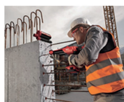
Wandverlenging met overlappingslassen
